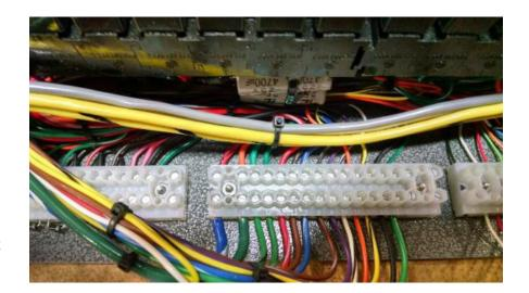
Wire the small gray 22-20 control cable to the 20 pole strip color for color. Crimp the provided 2 Awg / ¼" hole connectors on the black and red 2 Awg cables, red goes to the open "BAT" stud on the breaker and black goes to the ¼" ground stud with the lamp ground wires.
